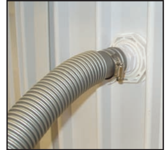
Figure 17 — Free end of hose attached to return
